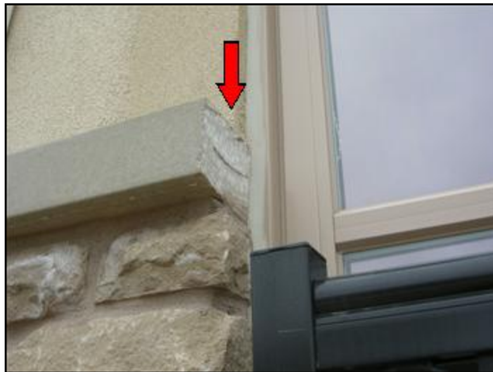
18. Exposed cut end of coping
